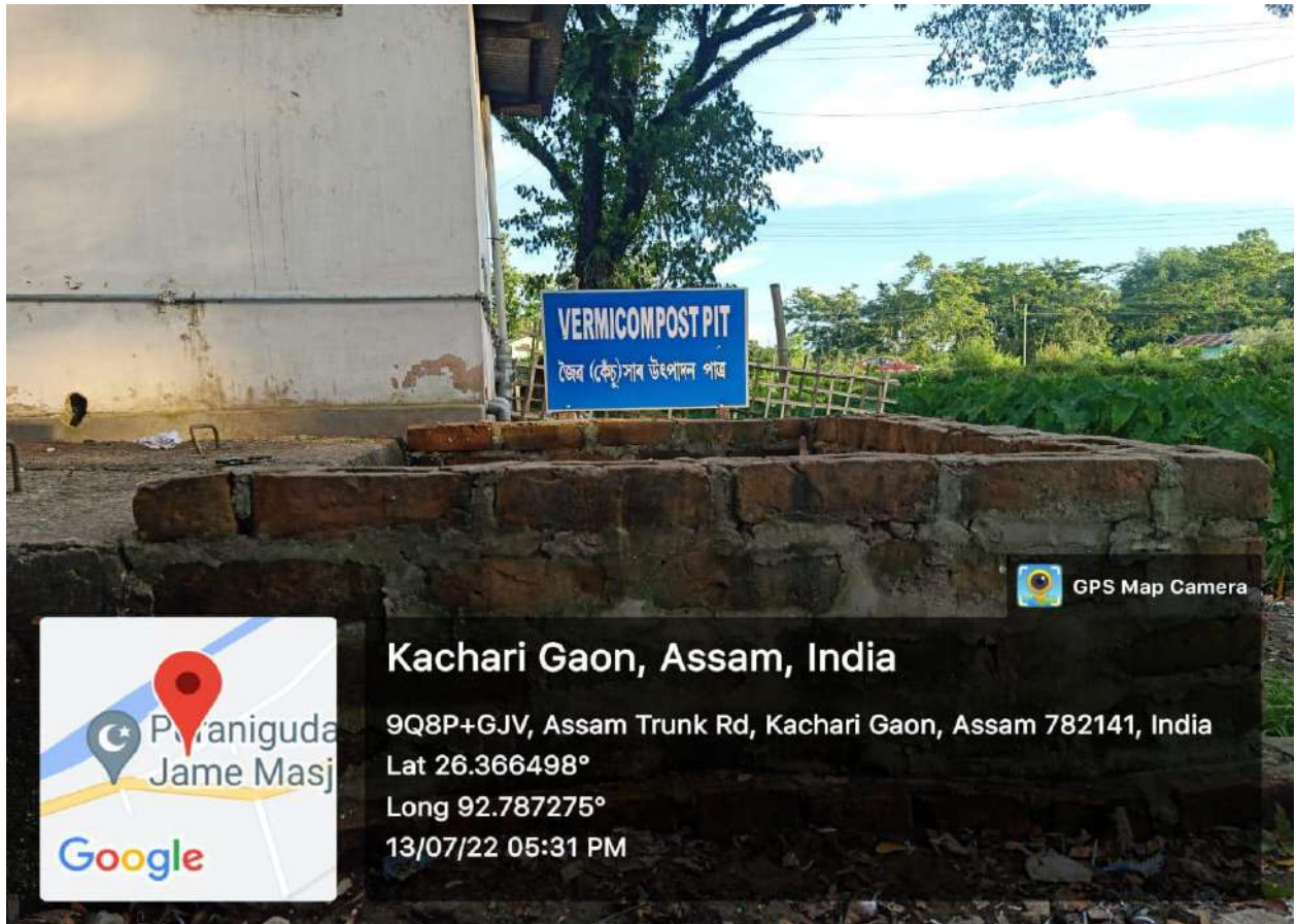
Degradable Waste Management: Photo of Vermicompost Pit
