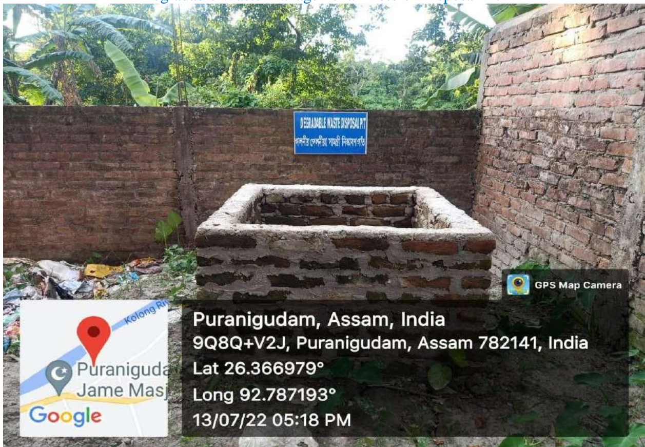
Degradable Waste Management: Photo of Disposal Pit inside the Girl's Hostel
